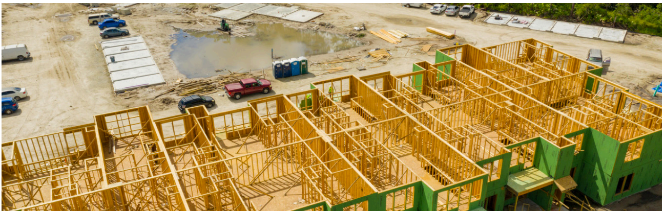
Photo: Construction site / Felixtm, Depositphotos
